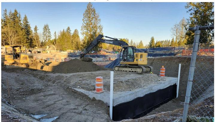
Construction crews work in late January on a large underground stormwater vault in the Sammamish Town Center area. The vault will have a capacity of more than 1.6 million gallons and is designed to help prevent flooding and reduce erosion in rivers and streams. It will be topped by open space.
